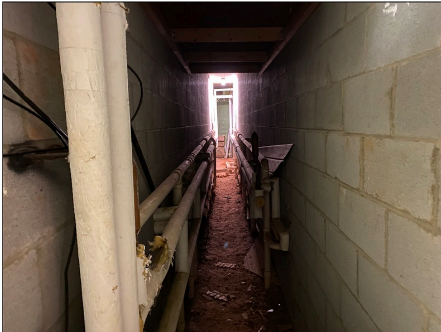
4 - View of the wall chase.
